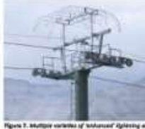
Figure 7. Multiple varieties of 'innovative' lightning arrestors.
